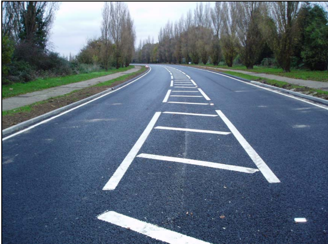
The Weeley Bypass, paved and open to traffic.
