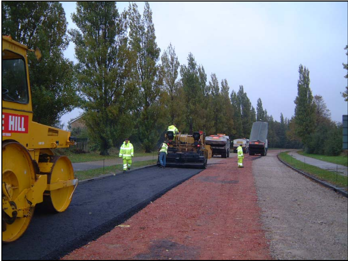
Paving operation on rubblised concrete surface.
