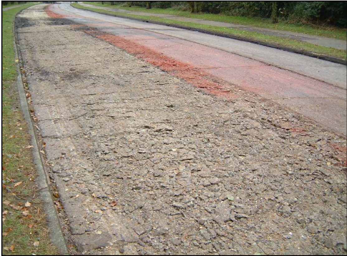
Close up of rubblised pavement
