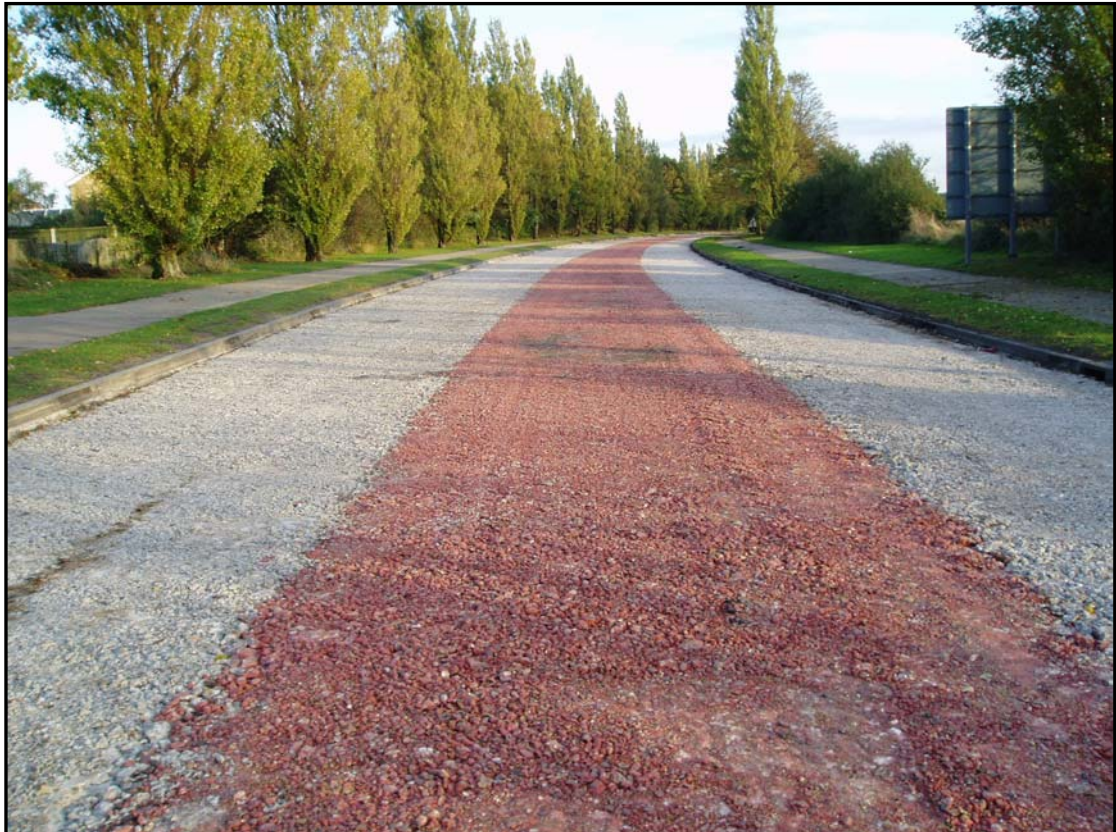
Rubblised concrete surface after compaction – ready for asphalt overlay.
