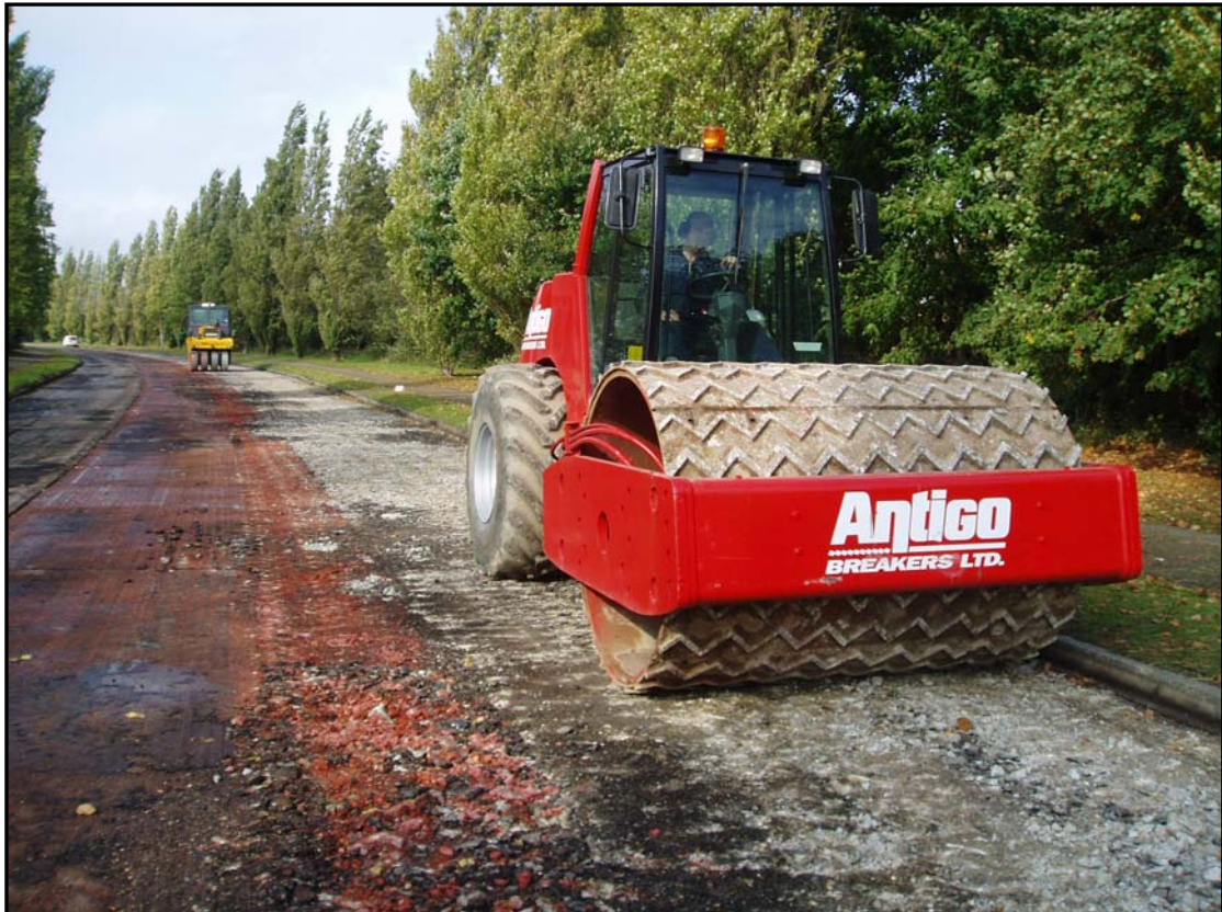
Grid roller reduces surface particle size and compacts rubblised concrete.
