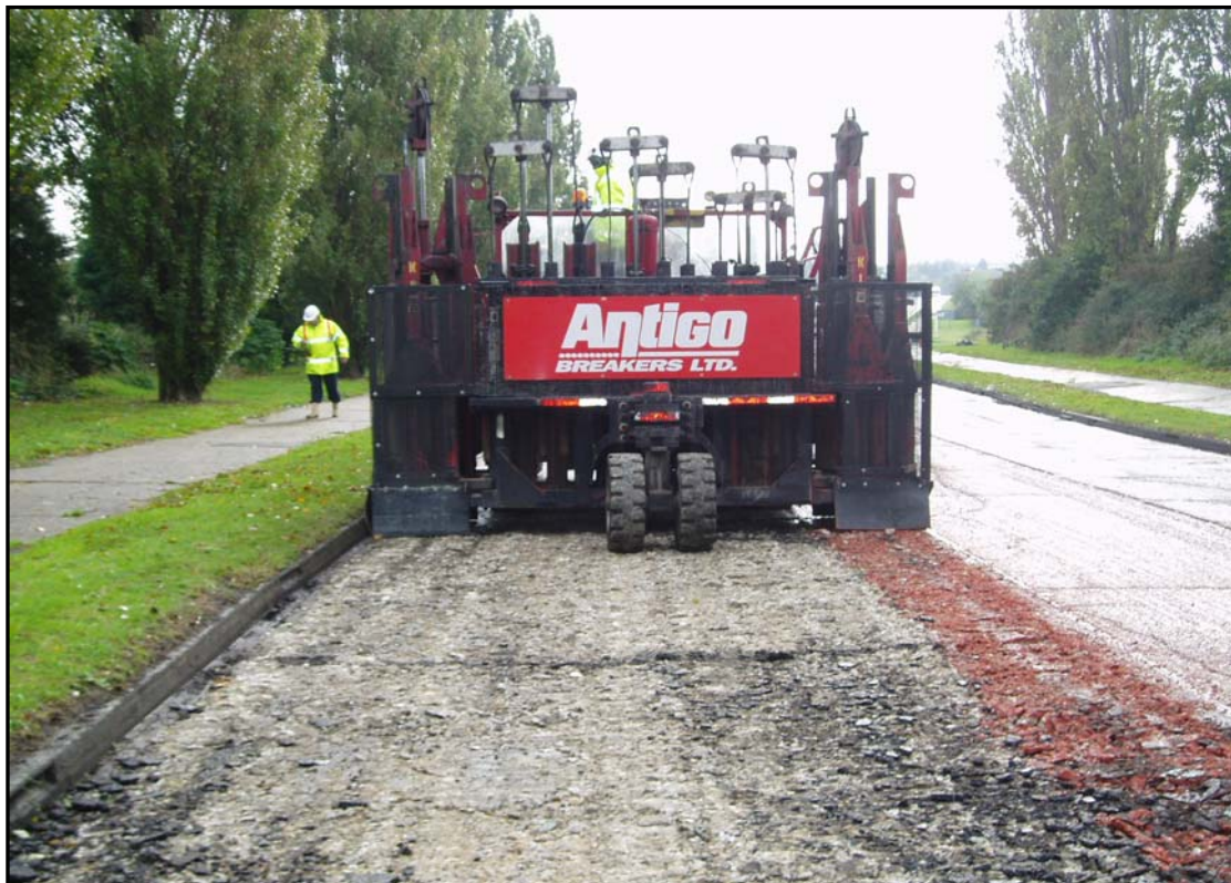
MHB Badger Breaker® rubblizing 1 lane after the removal of asphalt.
