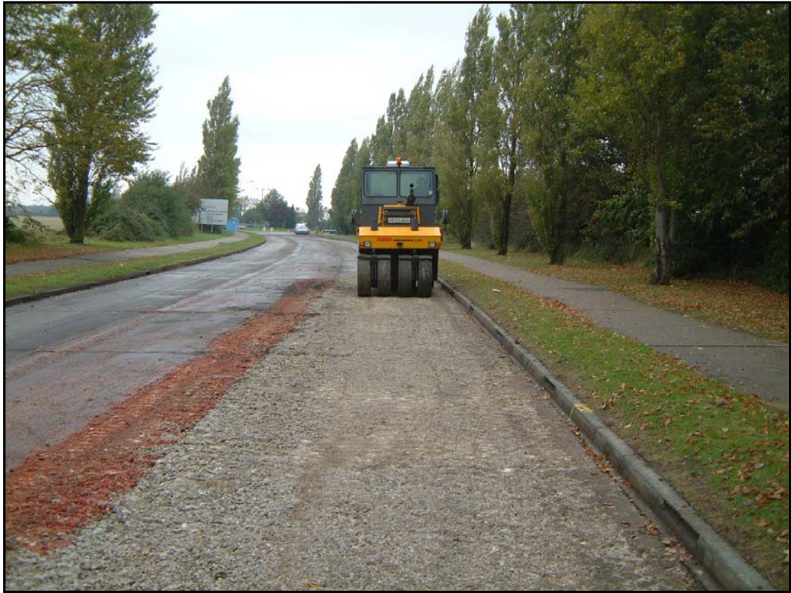
Pneumatic tyre roller completes compaction.
